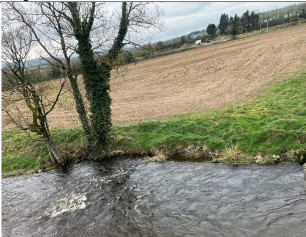
Photograph 3: Location of the new outfall, view from the bridge
